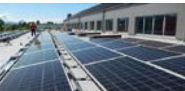
On a sunny day, it is expected that the panels will produce 143KWh, equal to approximately 9.4% of what the building uses. It is expected that the City will save approximately \$3,700 on annual power bills for the Civic Center and the building's carbon footprint will be reduced by 21.7 tons per year.
